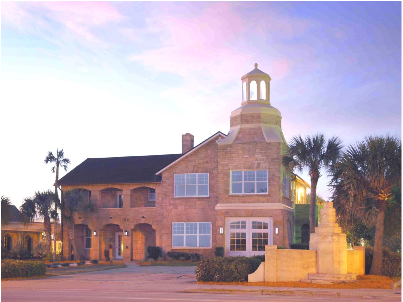
Fire House After Renovation in 2008
